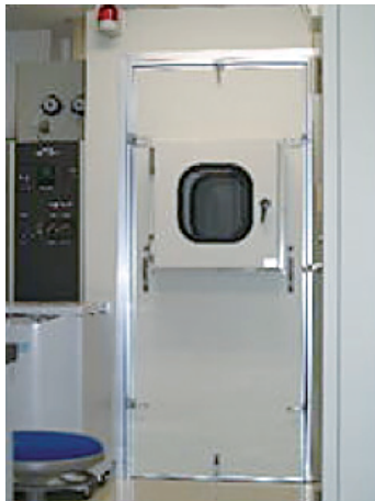
Window for handling preparations
