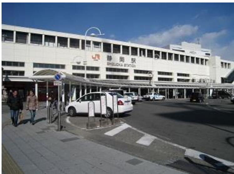
Panorama of Shizuoka Station (South side)
